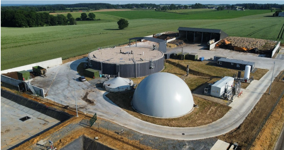
Picture: BIOGEST 140 Nm³/hr (41,857 MMBTU/year) PowerRing biomethane plant in Metha des Bosquets, FR
