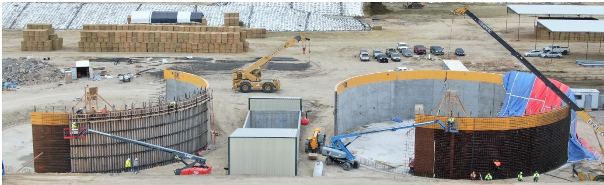
Picture (1): BIOGEST construction progress of 1 st biogas plant in Idaho, January 2021
